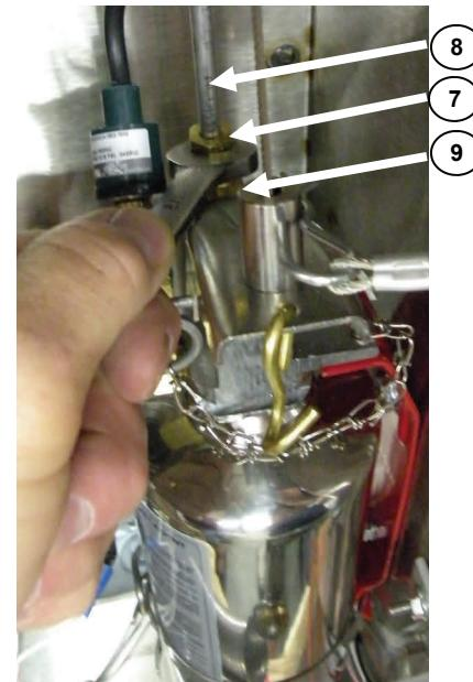
With a 1/2 inch open end wrench remove the 1/4 inch compression fitting (7) from the 1/4 inch tubing (8) at the tank adapter (9).
